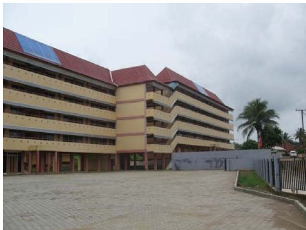
Public housing: Installation site for the Eco Tank
