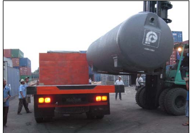
Eco Tank being transported to the project site
